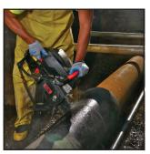
Safer to cut ductile iron
