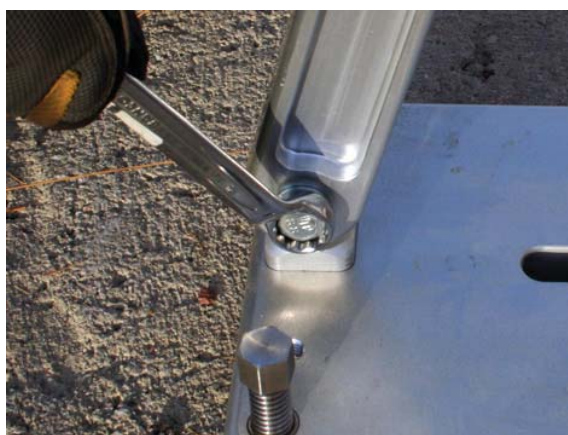
g. Tighten the lower bolt on the back brace.
