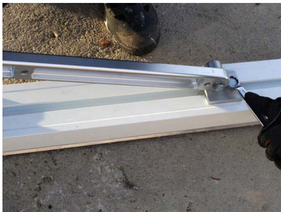
d. Tighten the upper bolt loosely.
