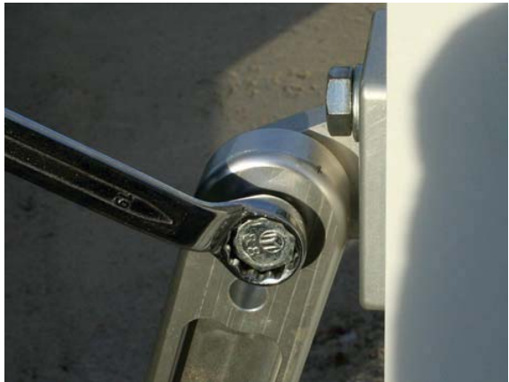
f. Next tighten the upper bolt on the back brace.
