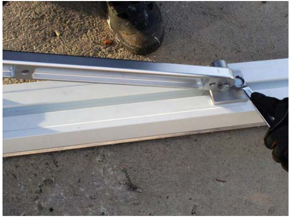
d. Tighten the upper bolt loosely.
