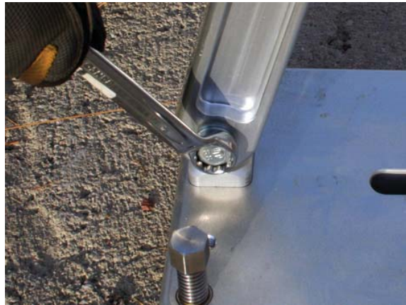
g. Tighten the lower bolt on the back brace.
