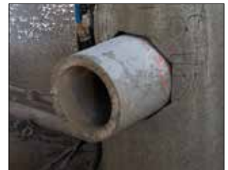
Pipe Splice - 5 linear feet
